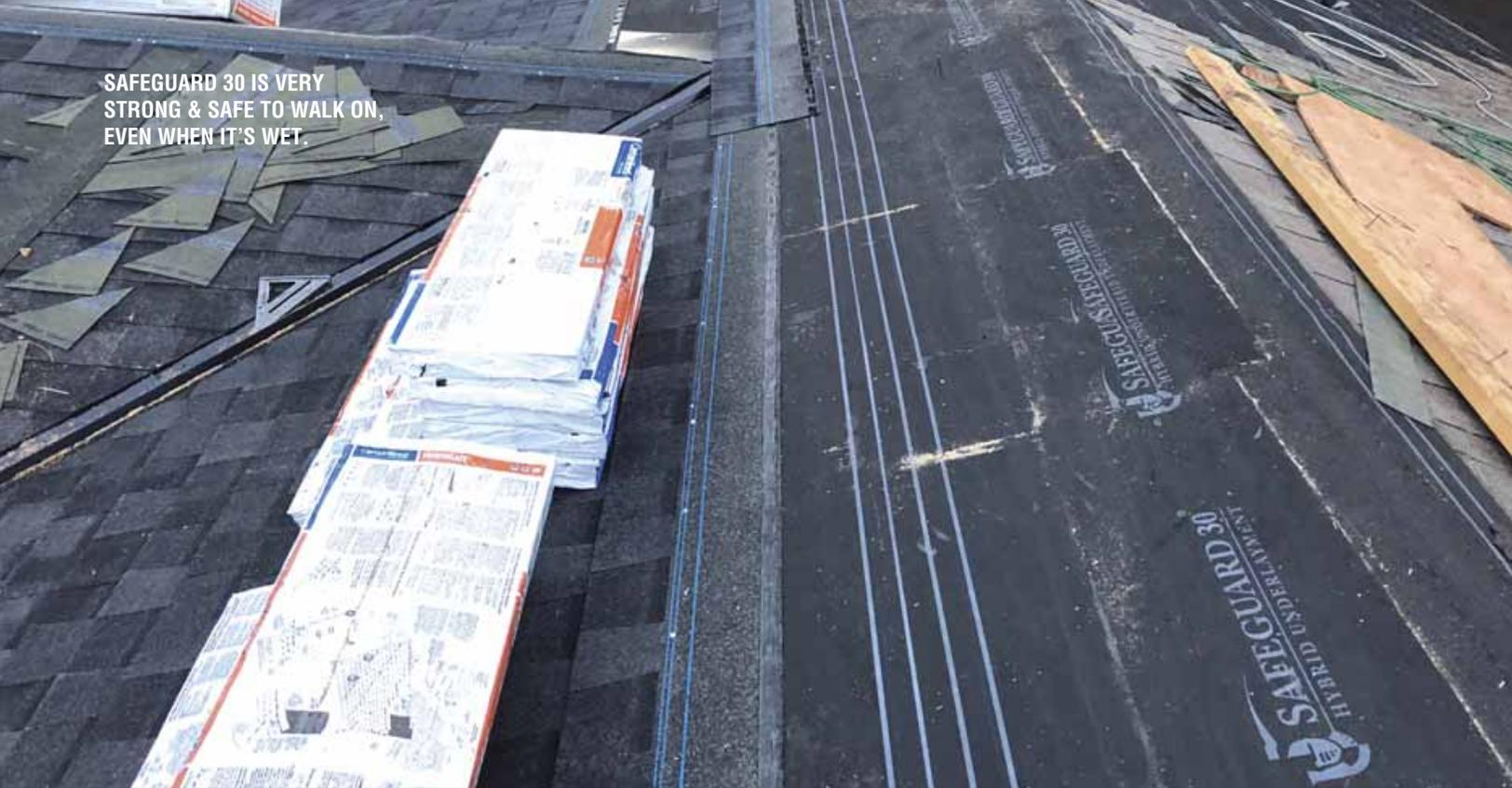
underlayments with a high-performance, nonwoven polyester reinforcement. The durability of Safeguard 30 hybrid underlayment allows it to hold fasteners better and provide better tear strength and puncture resistance than many other products on the market.
