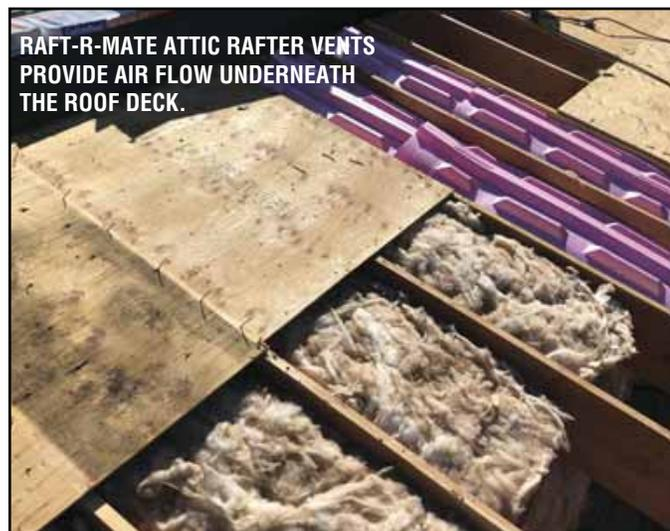
**RAFT-R-MATE ATTIC RAFTER VENTS PROVIDE AIR FLOW UNDERNEATH THE ROOF DECK.**
